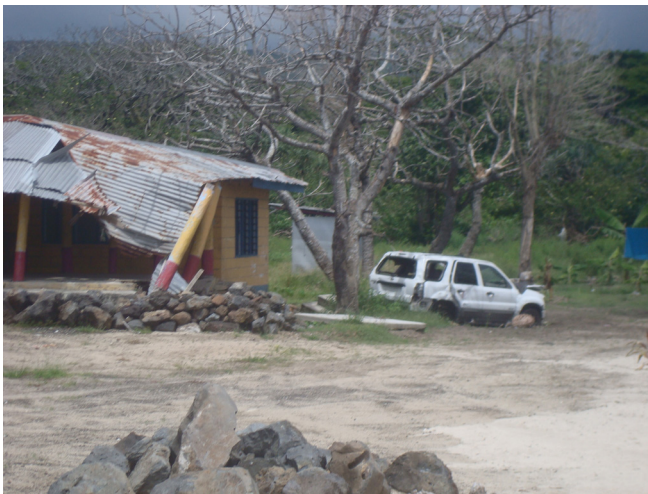
Damage from the 2009 tsunami. Credit: Helen Henry
