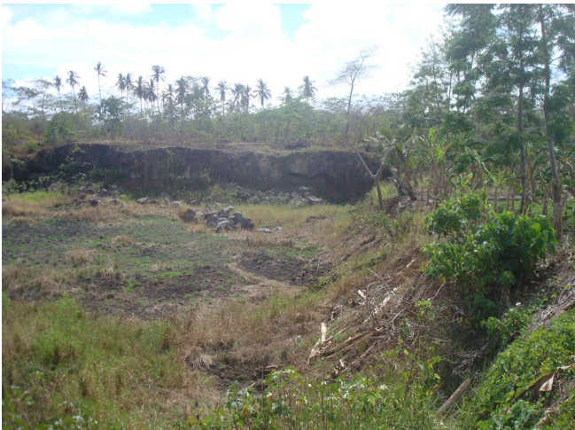
Rock quarry which provided material for coastal reclamation in 1997. The quarry has modified the flow of surface and ground water. In the wet season the quarry fills with water. When the impounded waters overflow there is serious flooding in neighbouring villages. In addition, two children have drowned in the flooded quarry. Credit: John Hay
