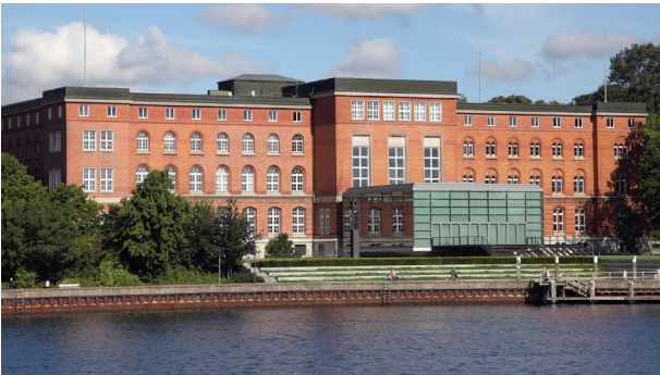
Different perspectives on the role of government between the United States and Europe affect how adaptation to climate change is conceived, funded, and implemented. Shown here is the government building of the German federal state of Schleswig-Holstein, located on the bank of the Baltic Sea. Credit: deli/fotolia
